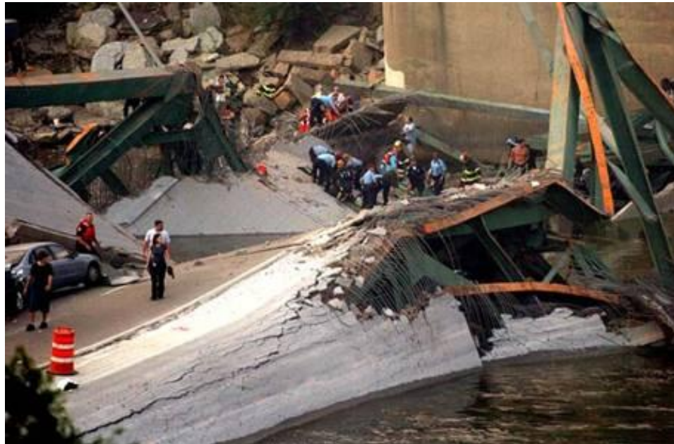
Looking at the collapse site on the northeast Minneapolis side of the river (across the river from downtown) showing police officers, firefighters, and civilians shortly after the collapse.
