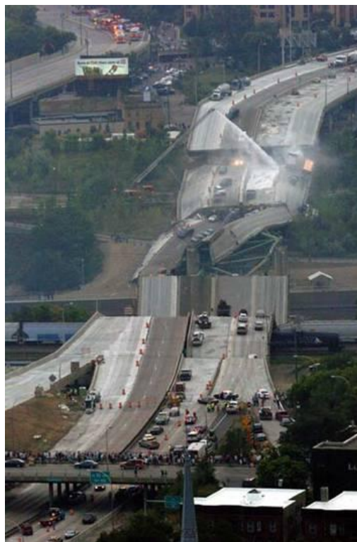
Overall view of the collapse site from the northeast Minneapolis side of the bridge. The standing bridge towards the bottom with all the people on it is University Avenue Southeast.
