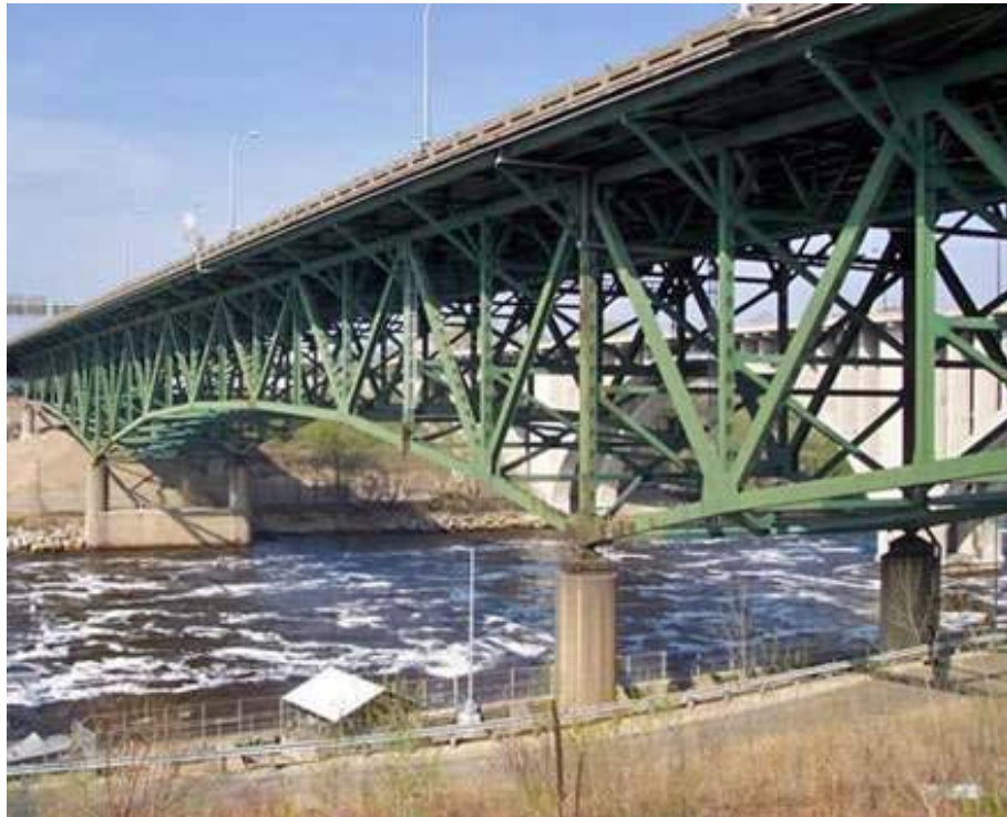
From the downtown Minneapolis side, showing the bridge before collapse and depicting the vertical distance from the bridge deck down to the river itself. (The river flows from left to right.)
