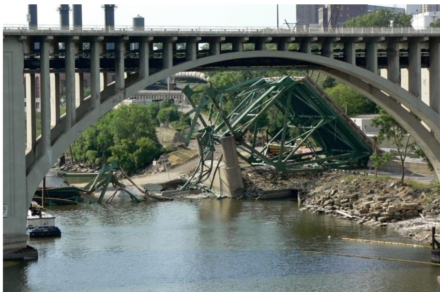
From the downtown Minneapolis side (but downriver from the above photo) showing how far the bridge fell and how far below road level the rescue work was being done. The standing bridge is the 10 th Avenue bridge, which ran parallel to the I-35W bridge as can be seen.
